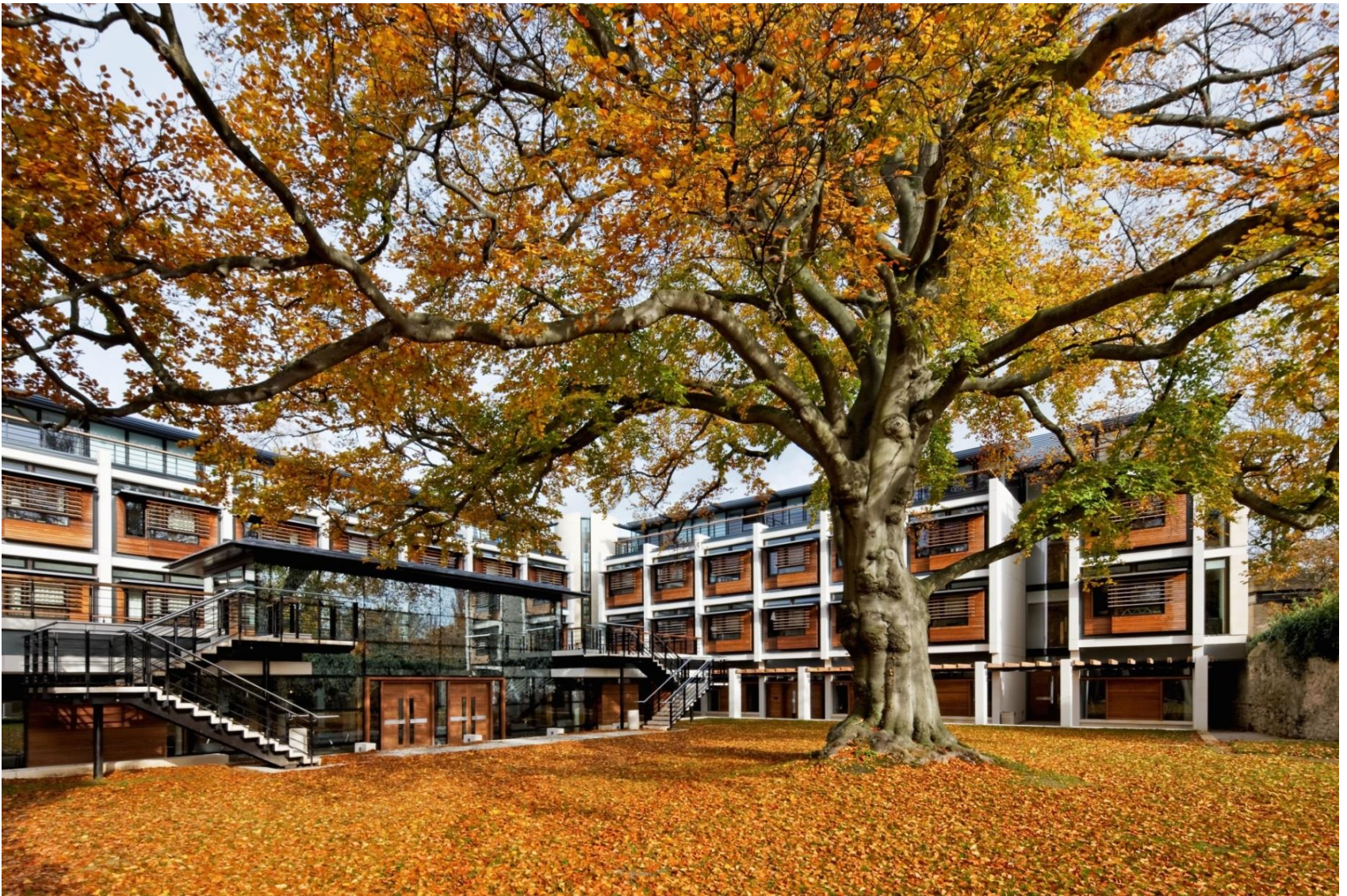
Community and identity: central quod (with tree) create a focus - St John's College Oxford, MJP Architects
